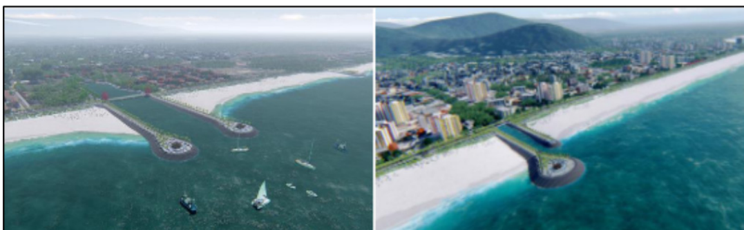
Figure 9. Current-Guides proposed for the artificial canal in Saint Etienne beach and Av. Paraná's canal (IAT, 2021).
