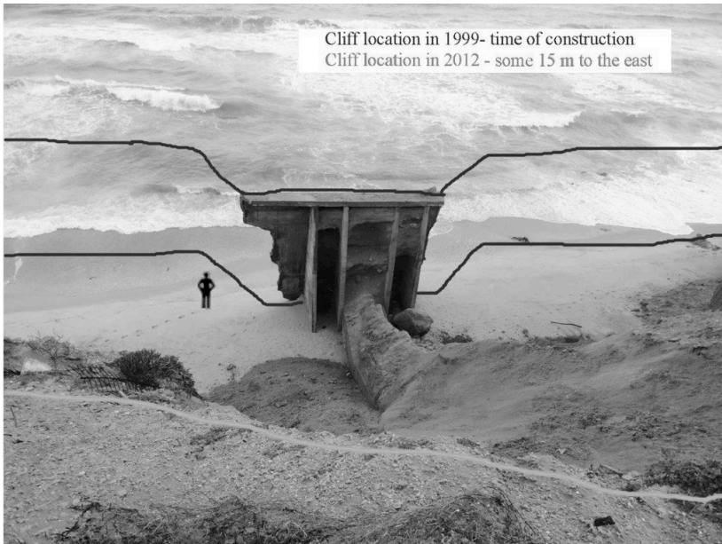
Fig. 12 - A sewer outlet in Ashkelon North, demonstrating the cliff retreat of 1 m yearly. The black lines depicts the location of the coastal cliff in 1999, the bright line indicates the present cliff edge (E.G.).
